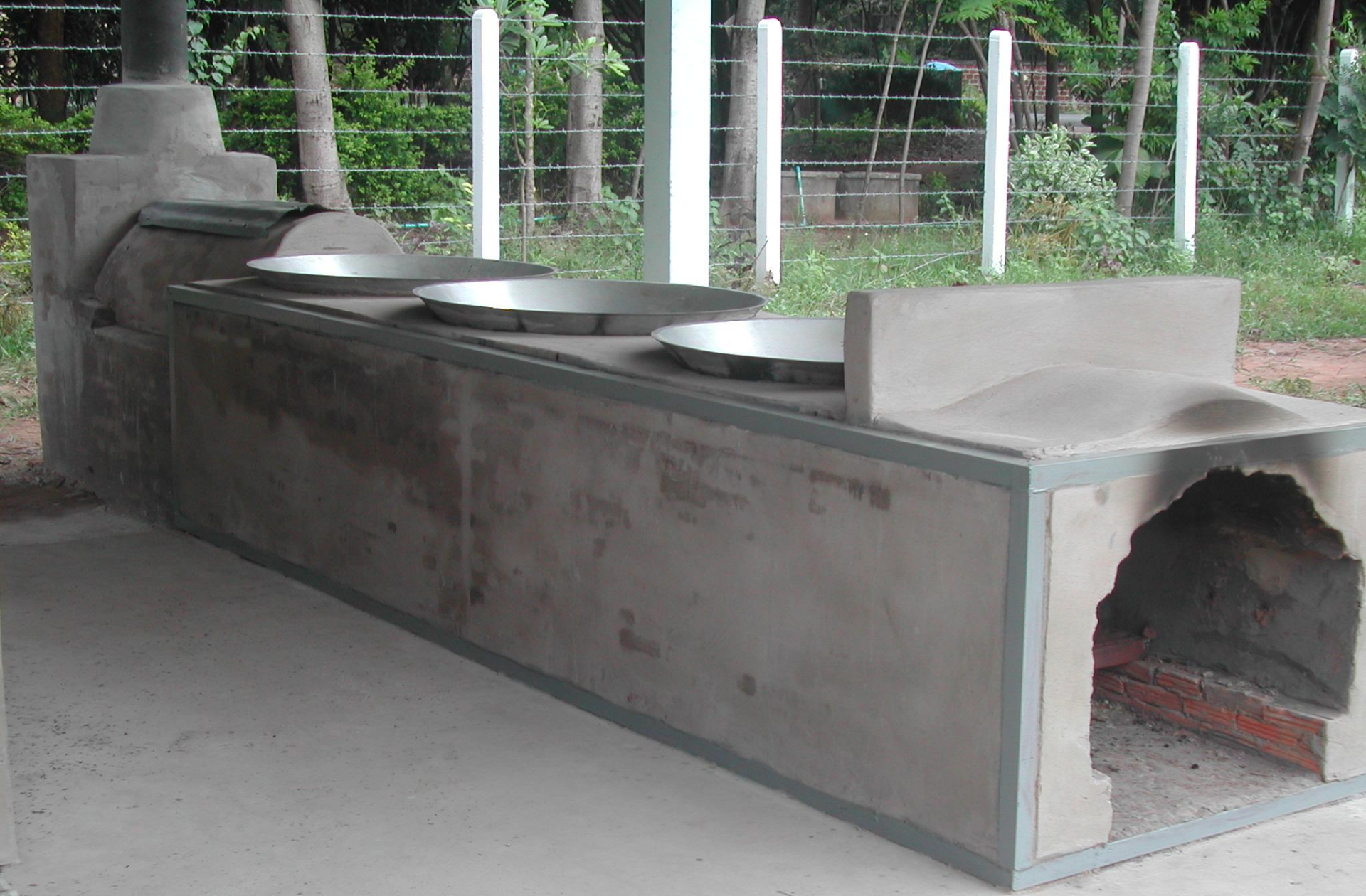
High Efficiency Biomass combustor for rural cottage industry
